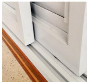
Shutterguard tracks butt neatly together to eliminate gaps.
